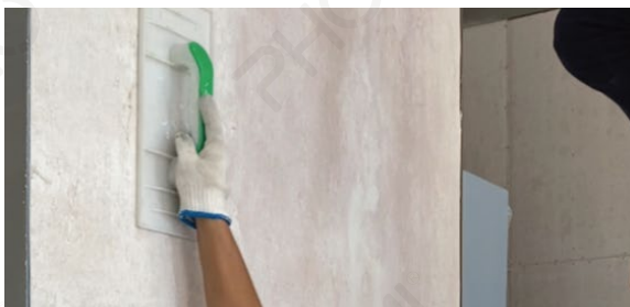
5.Compaction with board and guiding ruler
