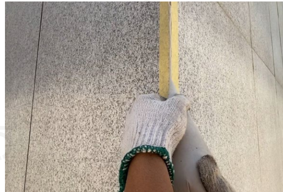
2. Caulk with a triangle bag of caulk
