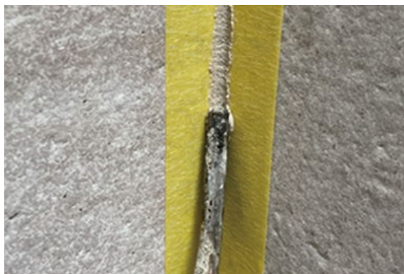
3. When the caulking agent is semi-dry, use the pointing strip with the same seam specification for pointing
