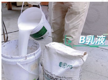
1.pour emulsion B into the barrel
