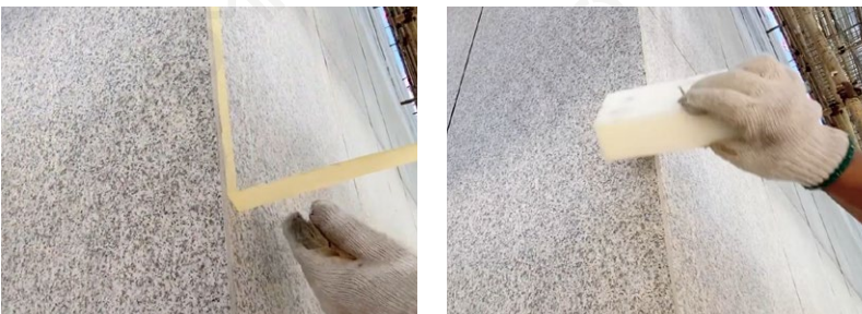
4.Tear off masking paper 5.Clean
