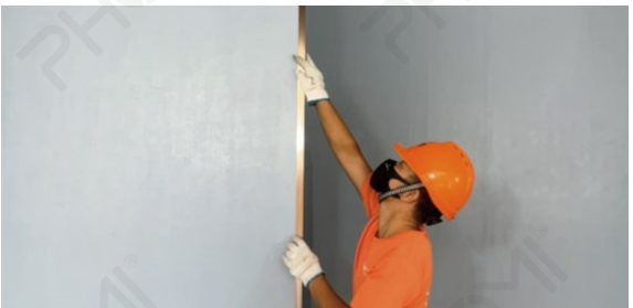
2.Stick the metal edge strips in external angle
