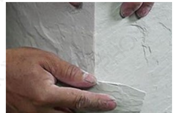
4. After the pulp dries, use a grinding wheel or the same color product to polish the corner to make it smoother.
