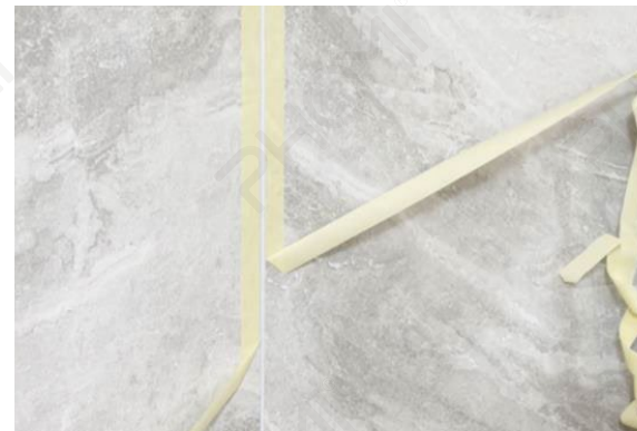
4. Tear off the masking paper
