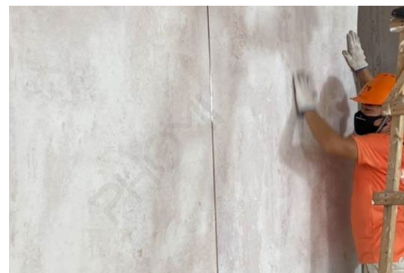
2. Paste the other side of the product along the decorative seam strip.
