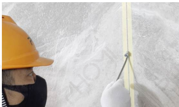
4.Caulk and Grout [1]
